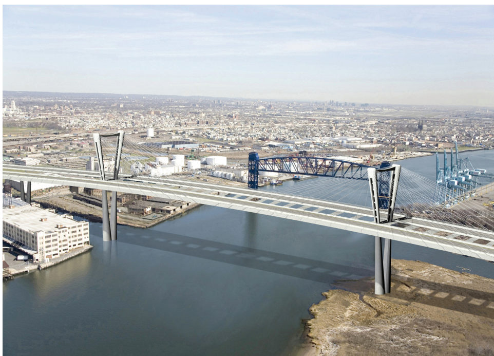
Goethals Bridge Replacement
