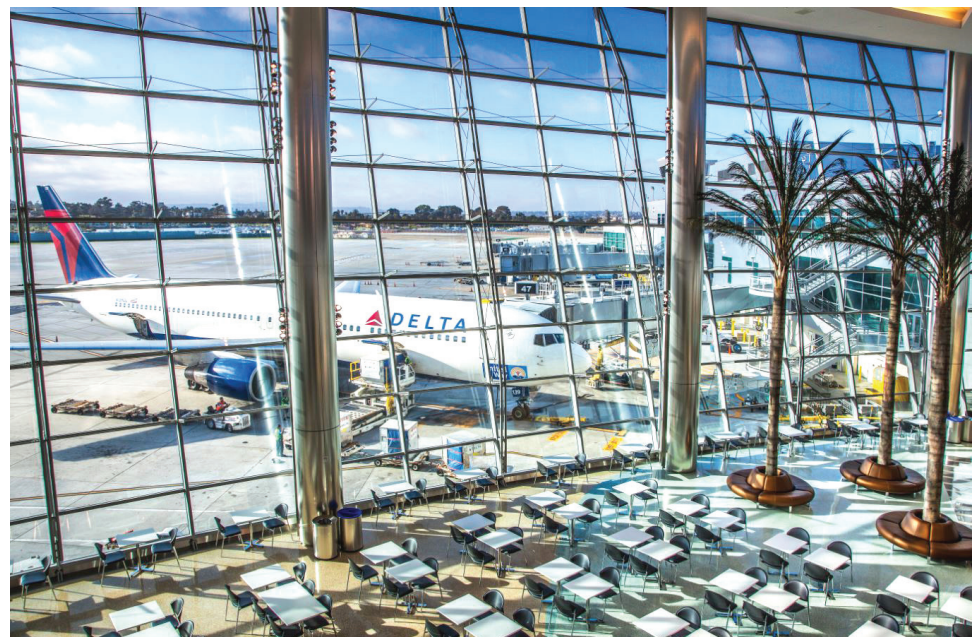
The San Diego International Airport Terminal 2 Building and Airside Expansion Project has been named as Best of the Best Projects winner for 2014 by Engineering News-Record.
